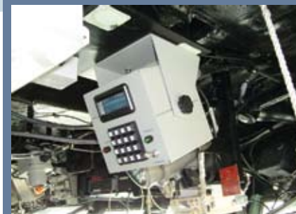
(top) Bottom view of the Ursa Navigator mounted in the old WRN-6 location (bottom) Remote installed to the old control indicator mount
