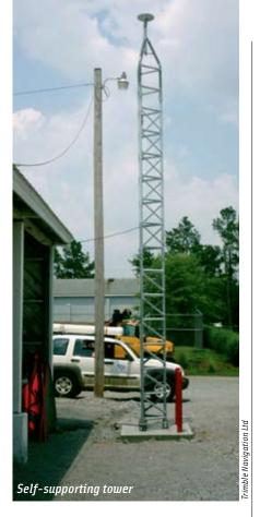
As a result of these criteria, many of the sites were located at South Carolina Department of Transportation (SCDoT) facilities. SCGS and SCDoT servers are located on the state Internet backbone and connected to each other by a virtual private network (VPN). At those sites where a suitable structure was not available, specially designed steel towers were erected as seen in the accompanying photograph.
